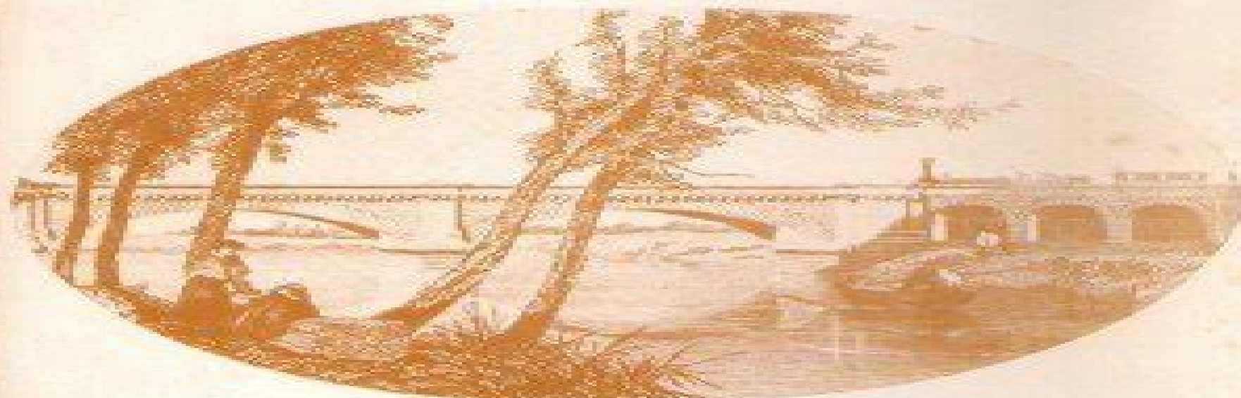
THE WARRINGTON VIADUCT seen from the River Mersey, and Mersey and Trent Canal
