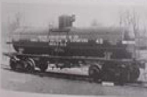
Southern Railway 1917 100000 gallon 40' 6" tank car built at 10' 10" car 1917 100000 gallon capacity 10' 10" car
