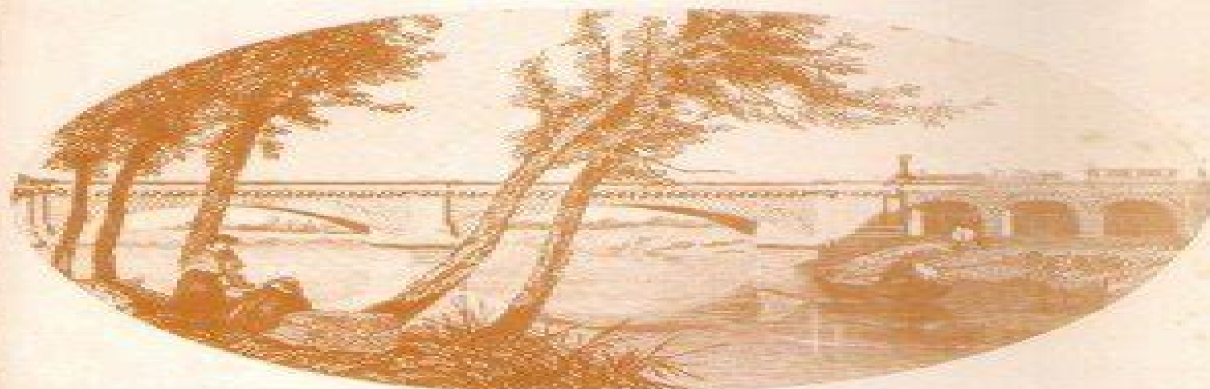
THE WARRINGTON VIADUCT over the River Mersey, and Mersey and Trent Canal
