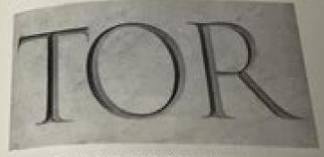
Fig. 31. Photograph of V-cut ridging in stone.
