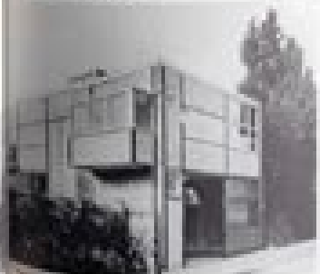
Fig. 7. The building, showing the main entrance.
