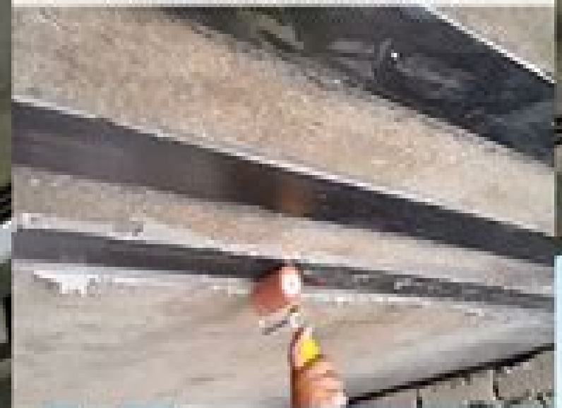
Carbon-FRP (CFRP) plates bonded to concrete surface with adhesive
